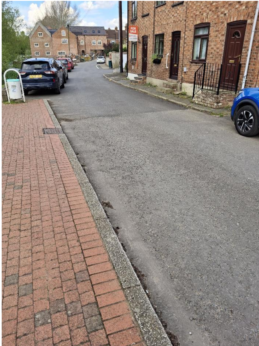
(Photograph 10.1 – Watermill Road; facing north-east)
