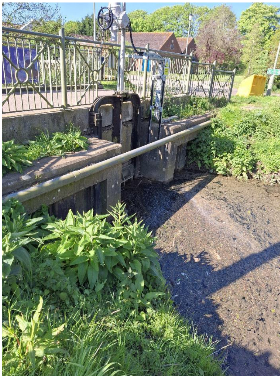
(Photograph 6.1 – Swimming Baths Sluice over the Old River Bain, with Horncastle Swimming Pool & Lifestyle Fitness Suite to the rear; facing south-west)
