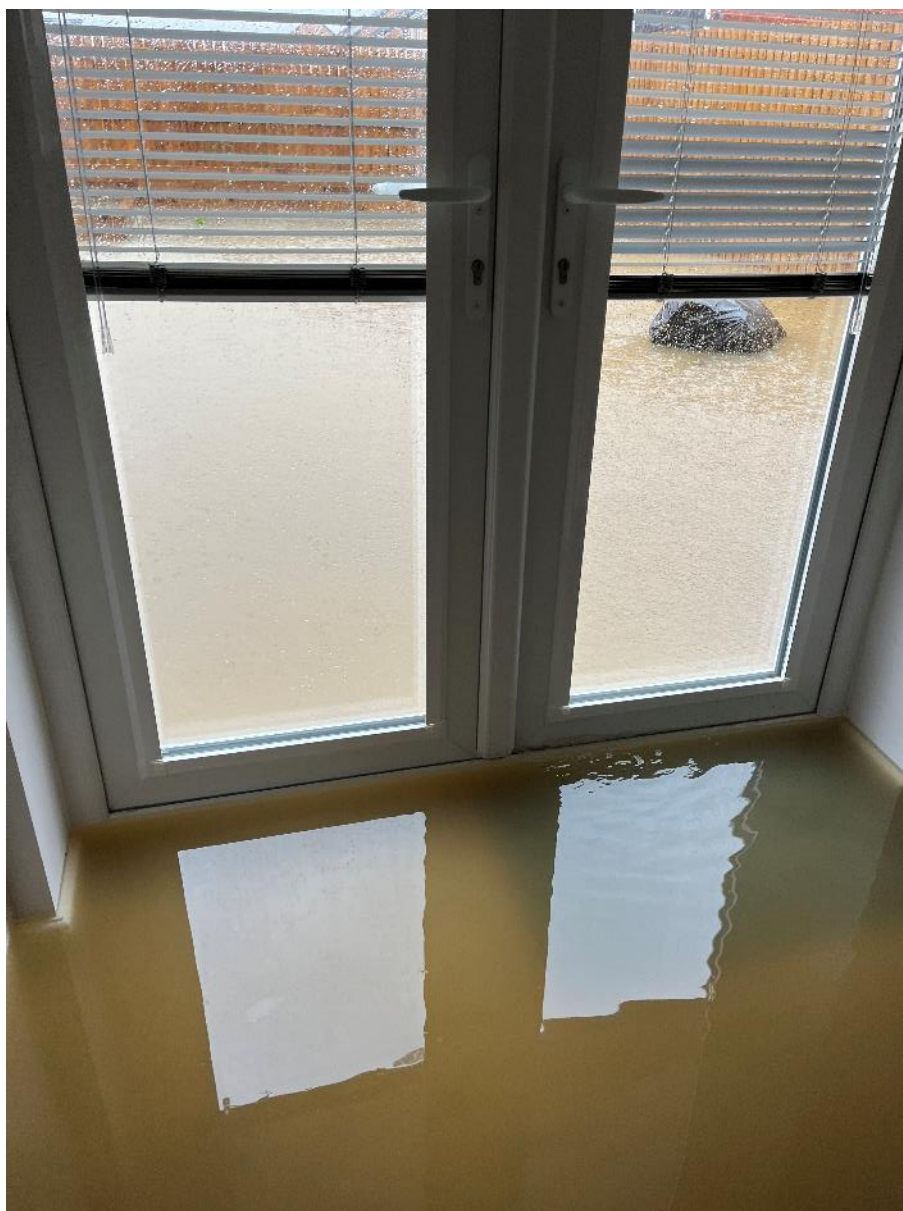
(Photograph 1.6 – Internal flooding at [REDACTED])
