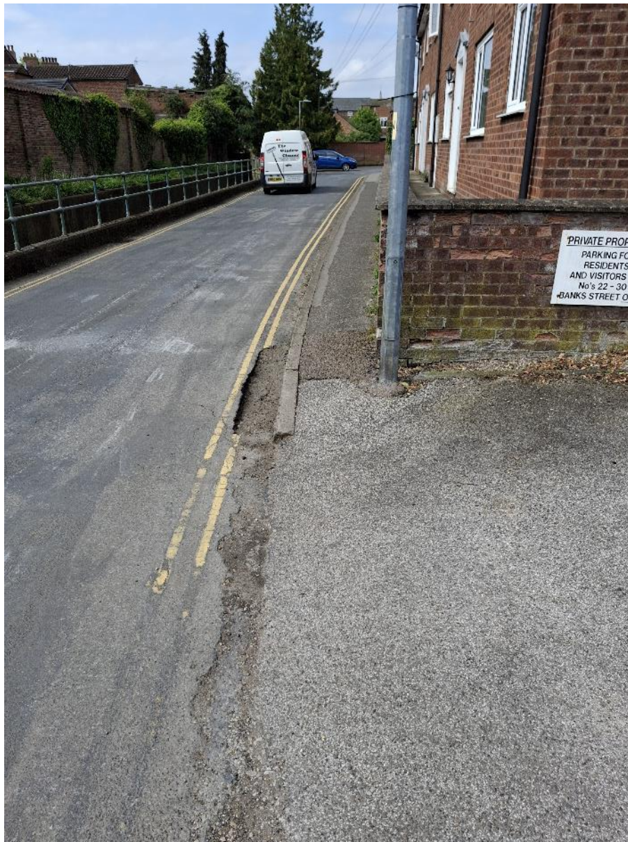
(Photograph 3.8 – Banks Street, with the River Waring on the left hand side; facing west)
