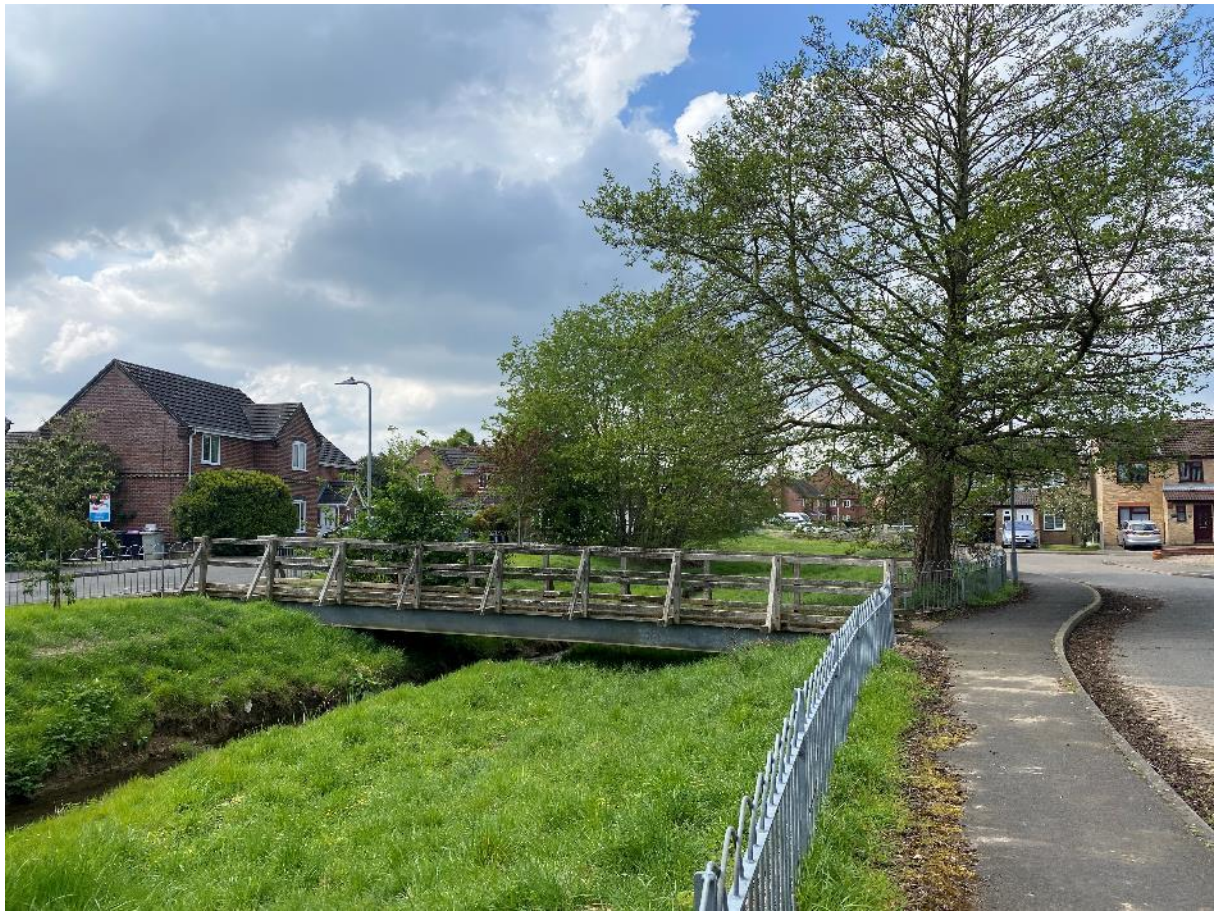
(Photograph 2.5 – The footbridge connecting Saxon Way and Lodington Court; facing west)
