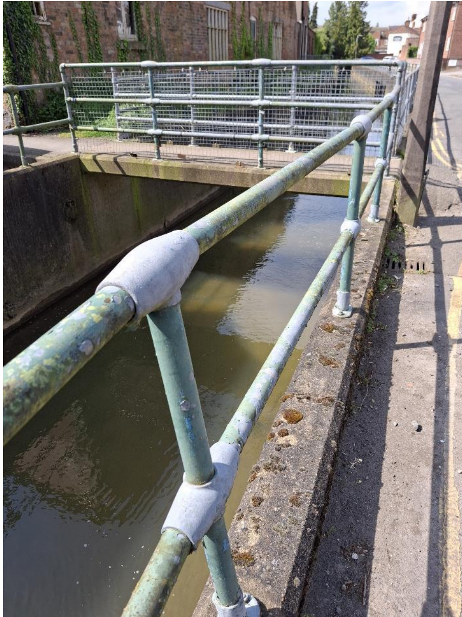
(Photograph 3.10 – Footbridge over the River Waring, connecting Banks Street and Francis Lane; facing west)
