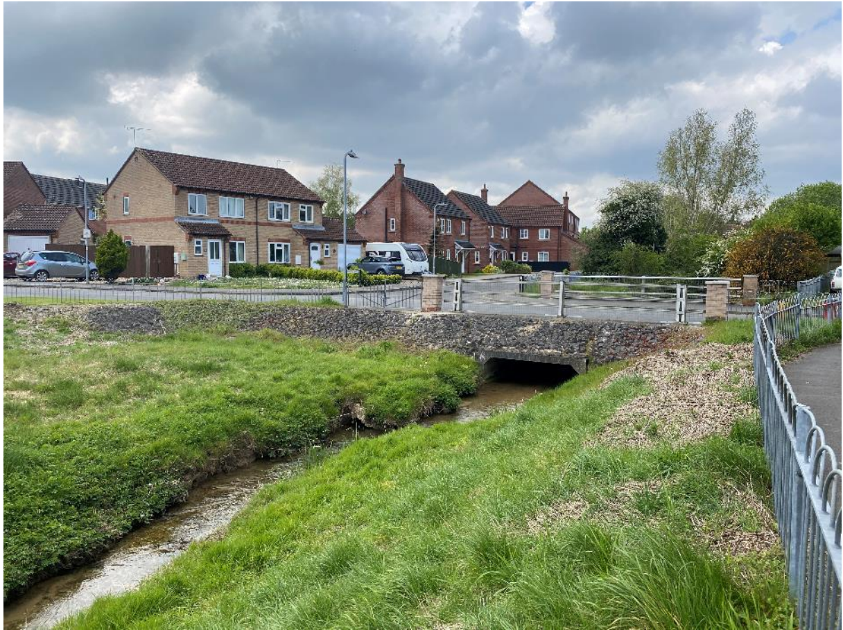
(Photograph 2.1 – The Thunker Drain, showing the bridge on Banovallum Gardens; facing south-west)
