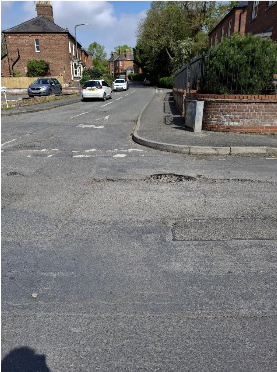
(Photograph 3.11 – Linden Road; facing north)
