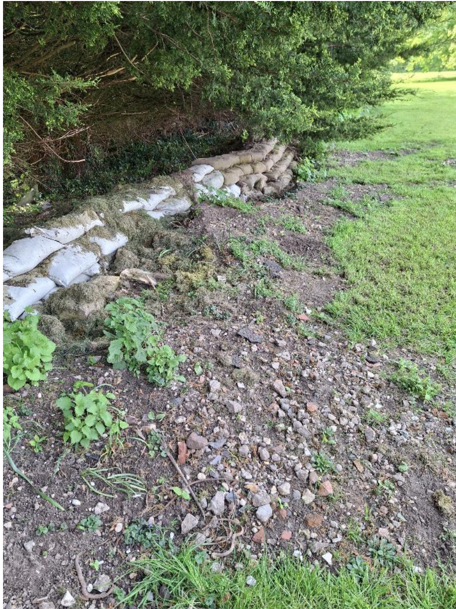
(Photograph 3.6 – Flood wall comprised of sandbags and concrete by the River Waring within the rear garden at [REDACTED]; facing south-west)
