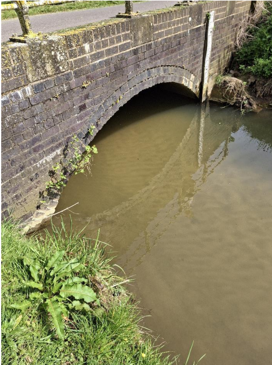
(Photograph 13.4 – Bridge over River Waring on low Toynton Road)
