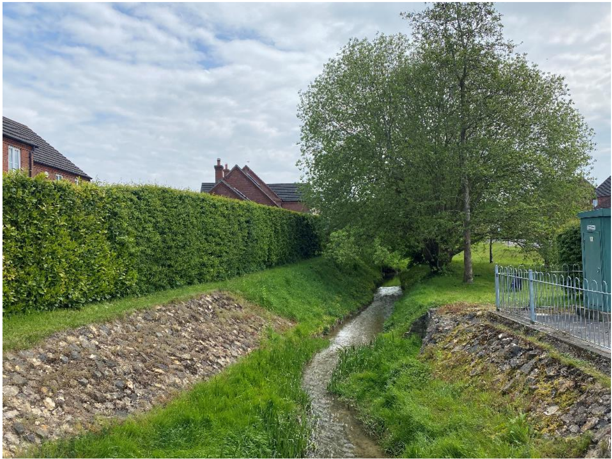
(Photograph 2.3 – Thunker Drain, as viewed from the bridge on Maltby Way in the westernmost area of the cluster. A pumping station can be seen on the right of the photograph; facing east)
