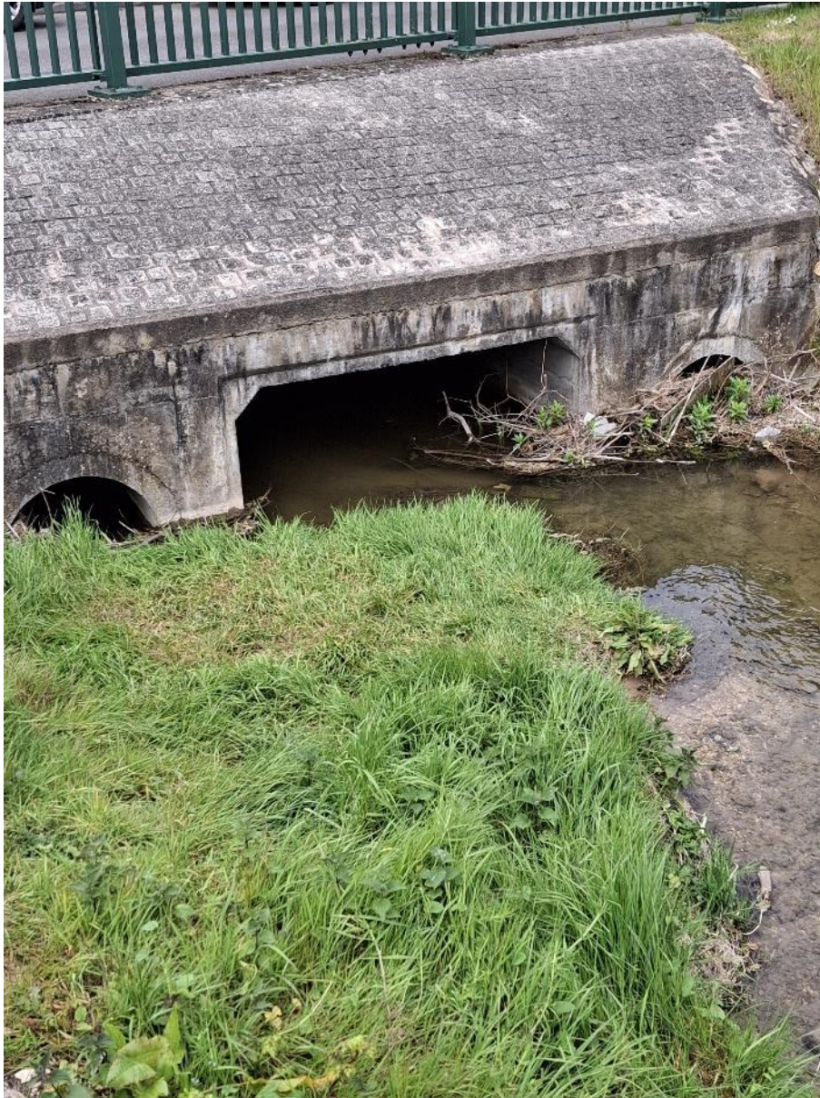
(Photograph 2.11 – Bridge at Maltby Way over the Thunker Drain; facing west)
