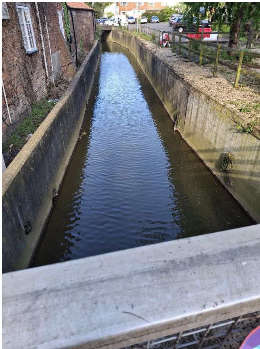
(Photograph 4.1 – Banks Street, with the River Waring on the left hand side; facing west)
